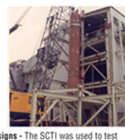
Evaluation of competing steam generator designs - The SCTI was used to test and compare competing engineering designs. The 75 megawatt steam generator on the left was designed by Atomics International while the similar sized unit on the right was designed by Babcock and Wilcox.
