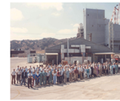
Experienced Staff – In 1974, approximately 1,800 people were involved with the engineering, development and testing of sodium components at SSFL. This photograph of ETEC staff was taken in 1986.
