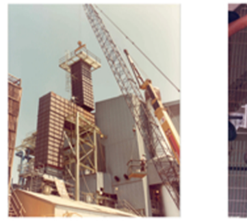
Natural Draft Heat Exchanger – This heat exchanger tested and engineering design intended to remove residual heat from a sodium system in the event of a sudden shutdown without using electricity.
