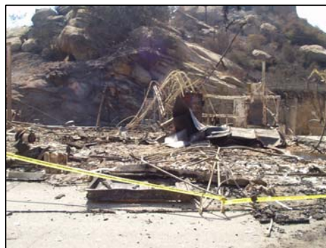
Fire damage at an inactive testing site
