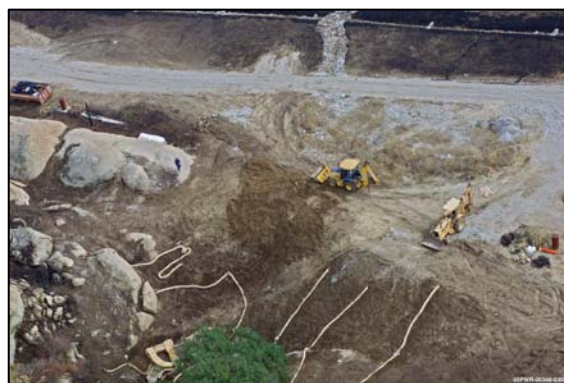
Installing erosion barriers in Area IV
