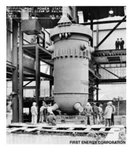
Shippingport Pressure Vessel Operational – 1957 (60 megawatt-electric)
