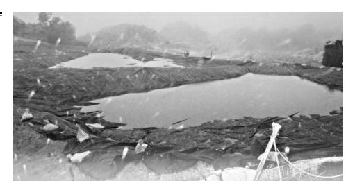
Throughout cleanup of the Former Sodium Disposal Facility, we have taken steps to keep contamination from leaving the site or entering the groundwater. These include covering the entire area with a waterproof material, constructing barriers in the two drainage channels to prevent soil from traveling down the channels, and re-directing surface water flow during rainy weather. These activities are performed during the rainy season and will continue until the cleanup of this facility is complete.
