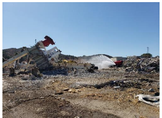
Sodium Pump Test Facility post-demolition dust suppression
