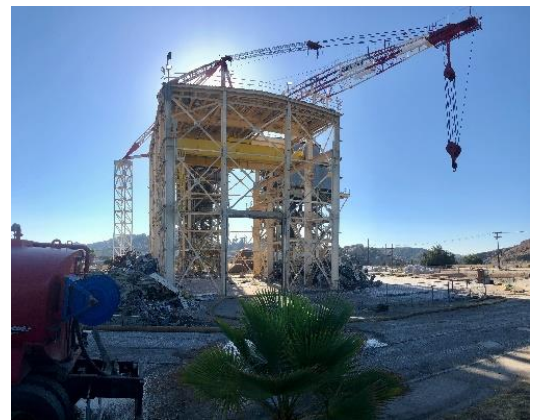
Sodium Pump Test Facility mid-demolition
